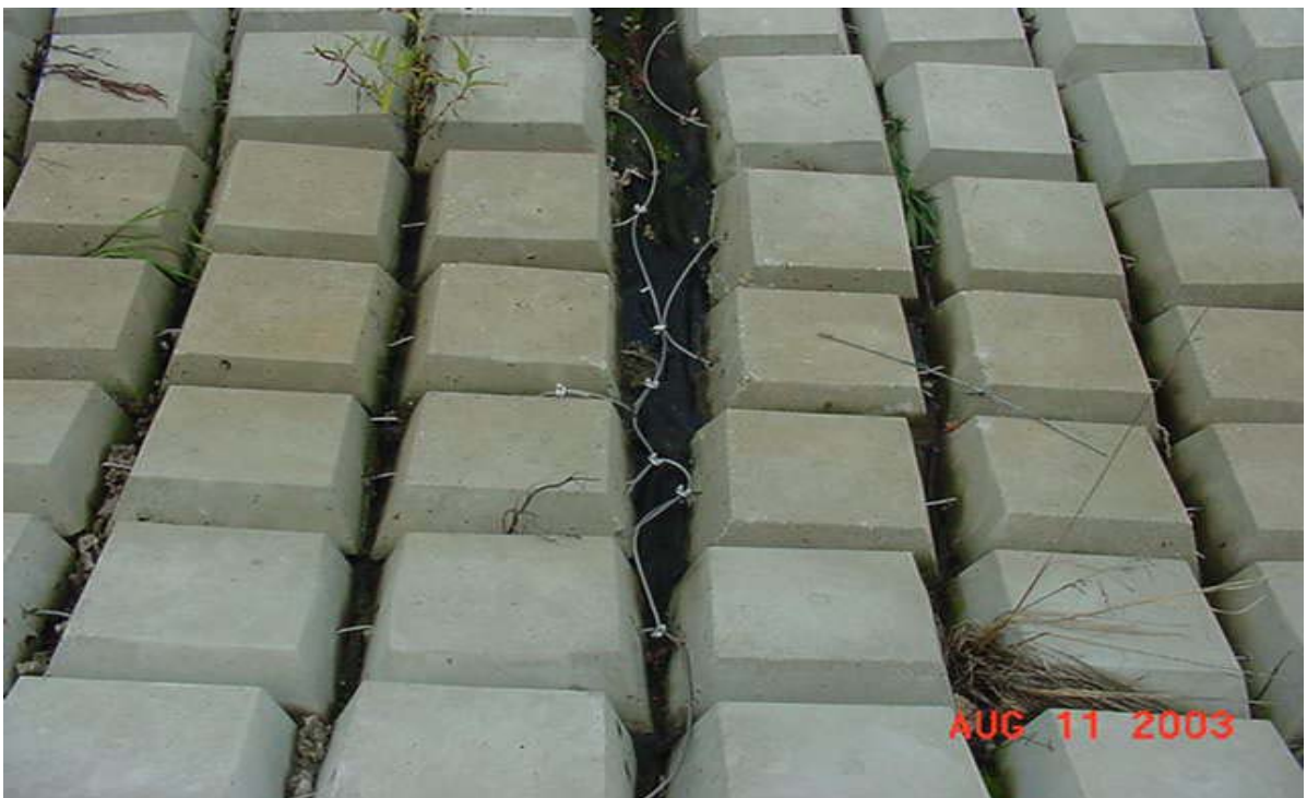
Photo 2 – Blocks positioned in place with clamps added
